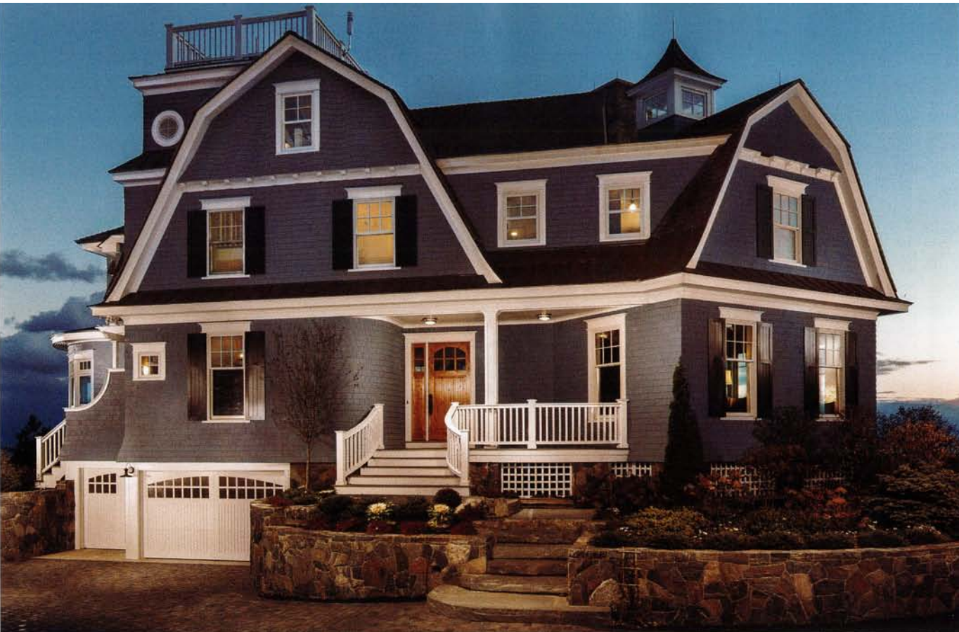
A front view of the traditional shingle-style cottage with gambrel roofs, a widow's walk, and porthole windows (above). "The massing of the house is broken up by the horizontal banding of the rooflines," says architect Brian Beaudette, who has offices in Kennebunk and Rangeley.
